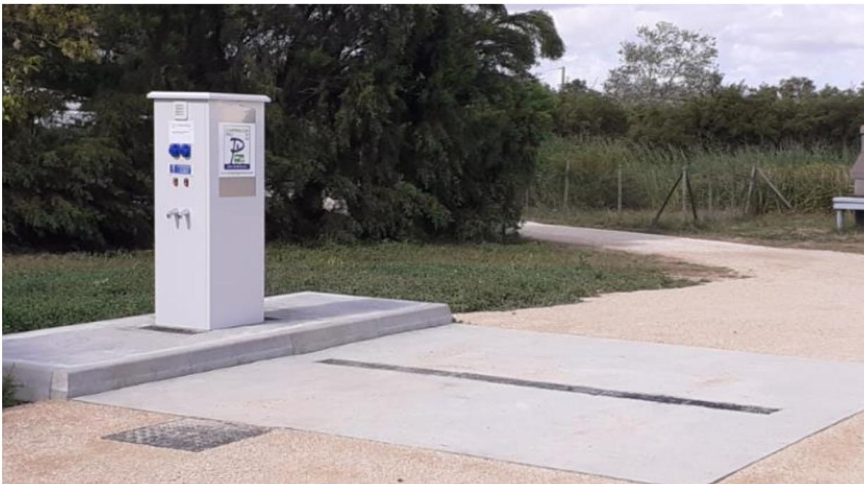
Cost: 3m channel drain, 3mx2m concrete slab
