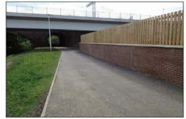
TYPICAL EXAMPLE OF BRICK FACED WALL (WATER OF LEITH, EDINBURGH)
