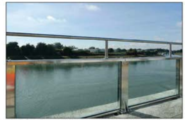
TYPICAL EXAMPLE OF GLASS WALL FLOOD BARRIER
