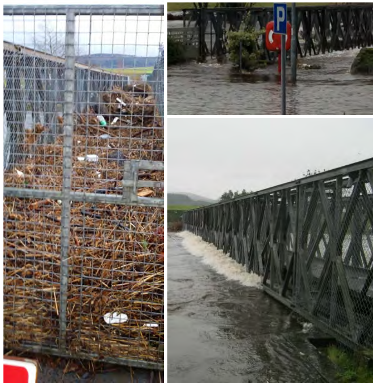
Figure 10-1: Old Sparling Bridge; debris building and flood waters backing up
