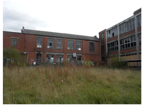
Former Power House Building to north
