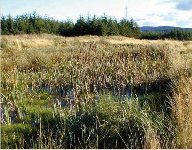
*As water filters through the roots and decaying plant material in this constructed wetland, toxic metals are removed. Craigenbay 1996. (Forestry Commission Scotland)*
