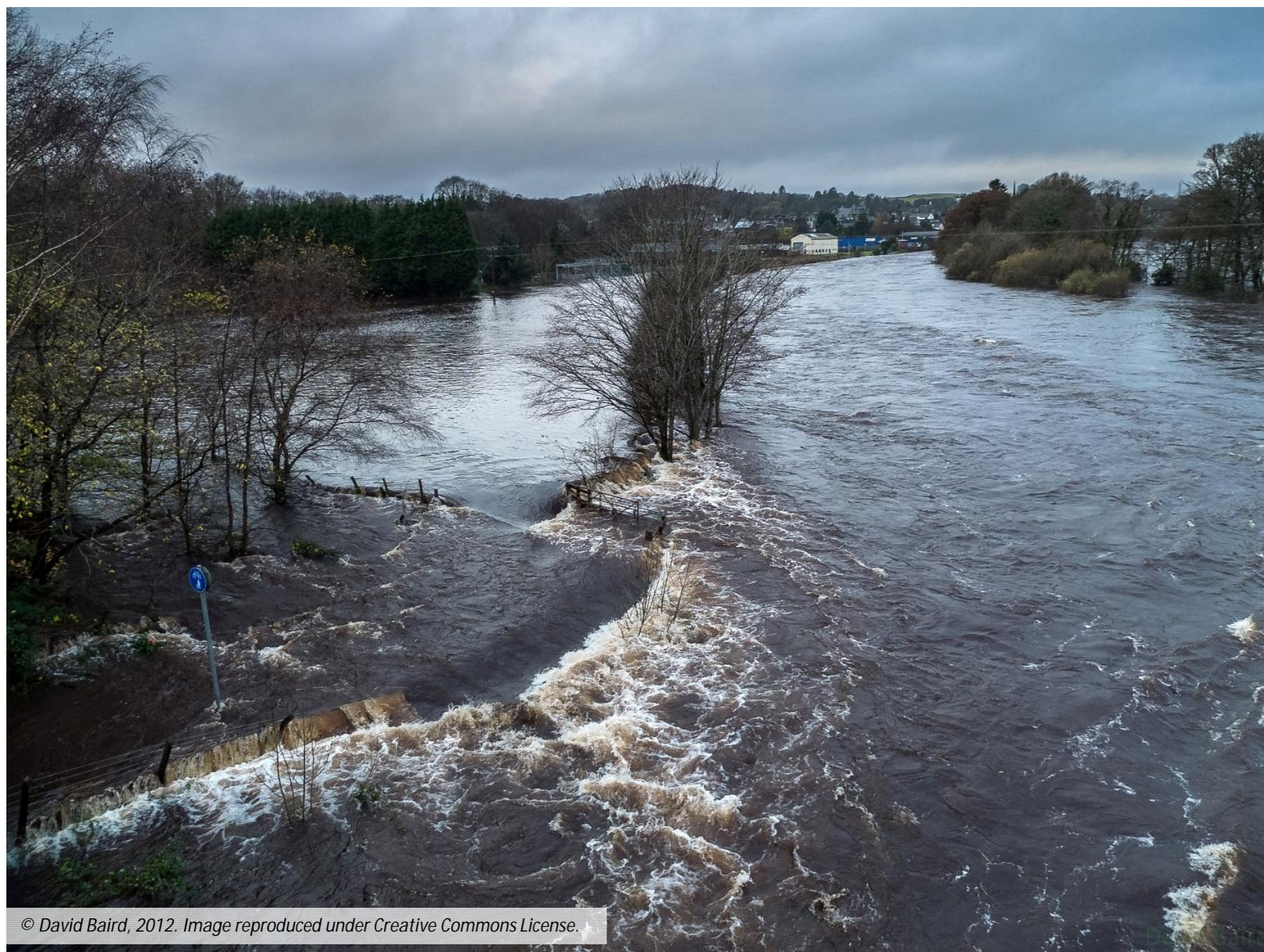
Figure 14-1: View from A75 Bridge During Flood (Looking Upstream)
