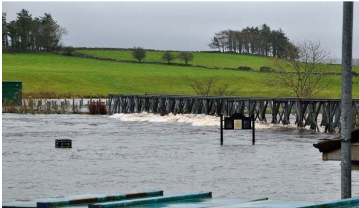
Photo – 24: Flooding at metal footbridge (Courtesy of Mark McKie via flickr.com)
