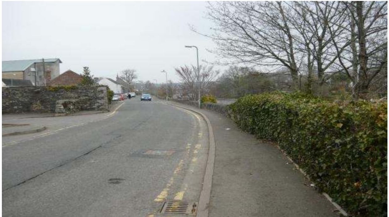
Photo – 11: Riverside Road – Upstream view taken a short distance upstream of the metal footbridge.
