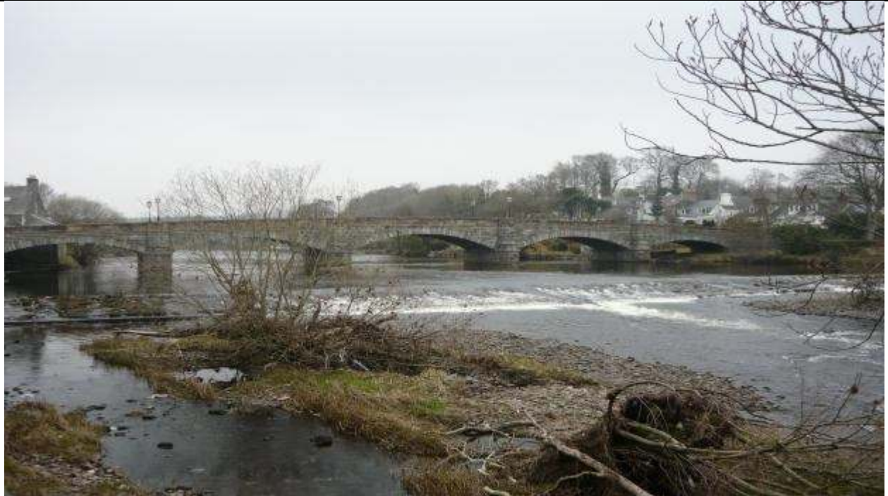
Photo – 10: River Cree – Upstream view of Main Bridge over Cree and masonry weir.
