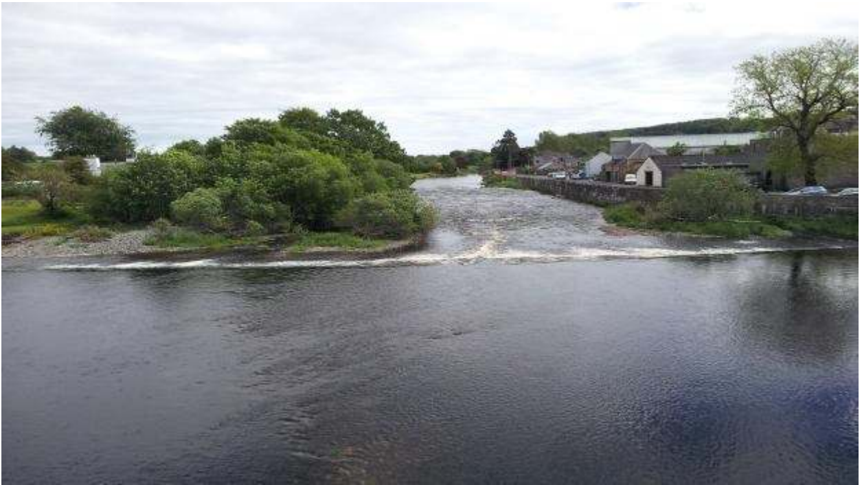
Photo – 7: River Cree – View of masonry weir and gravel berm taken from Main Cree Bridge.
