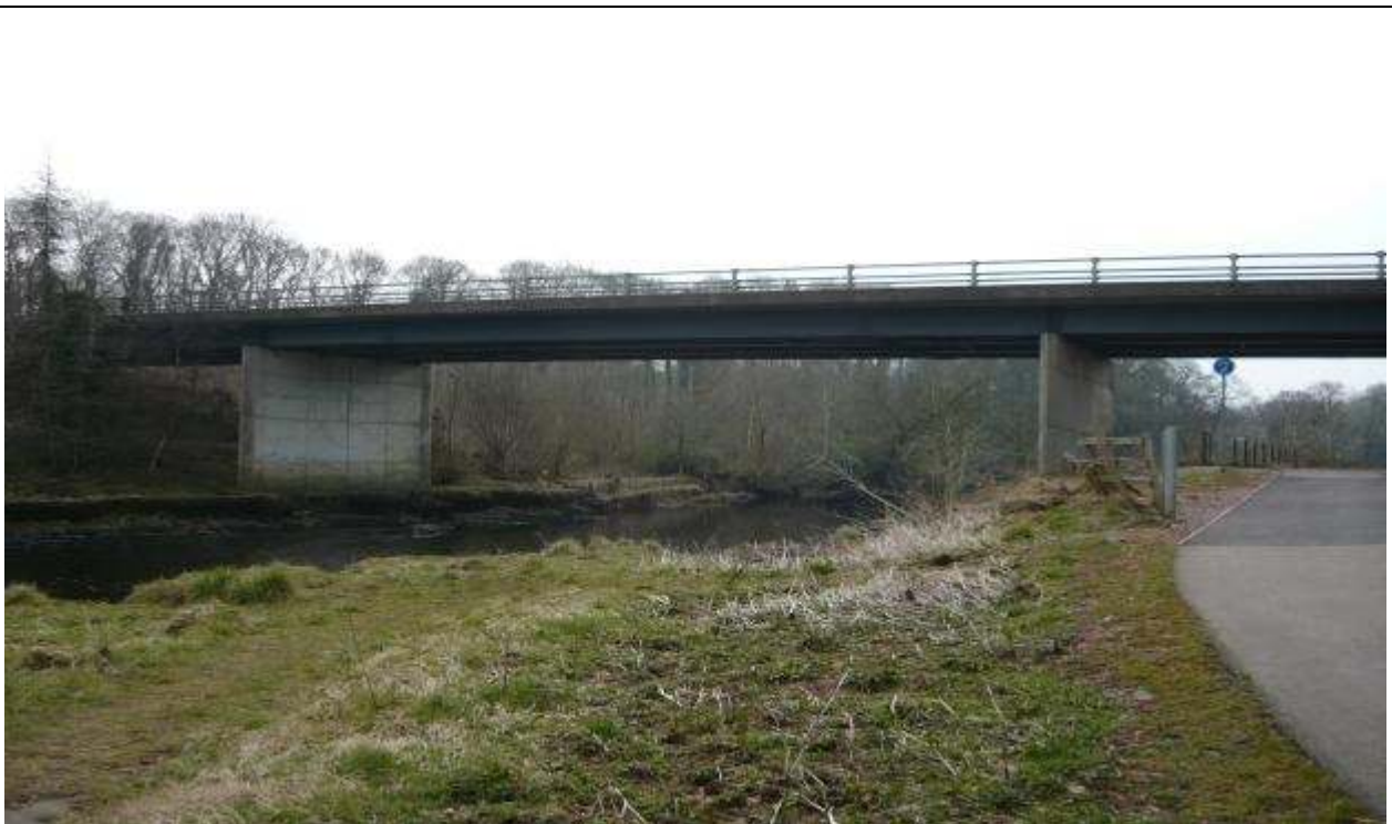
Photo – 15: River Cree – Upstream view of A75 road bridge
