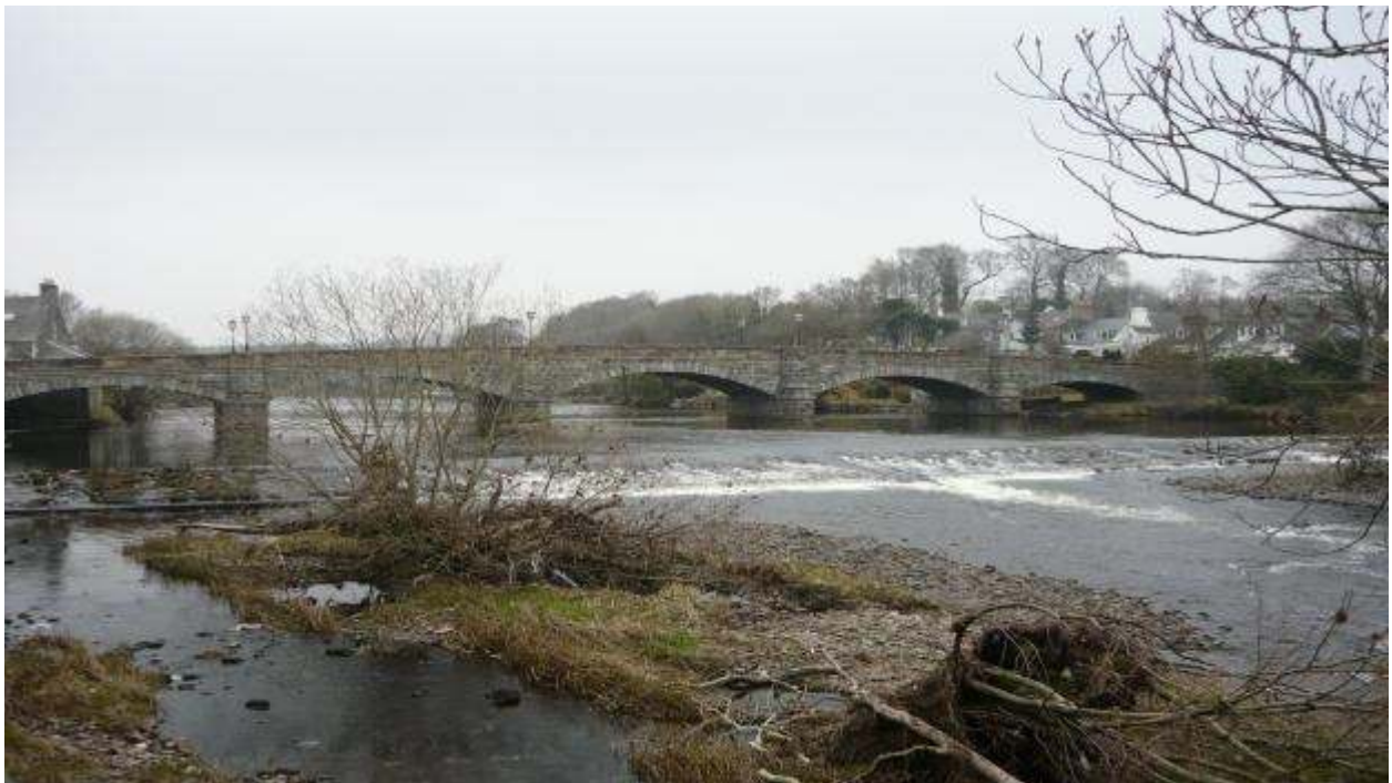
Photo – 6: River Cree – Upstream view of Main Bridge over Cree and masonry weir including western
