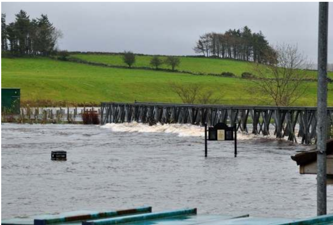
Photo 2: Metal footbridge during November 2012 event
