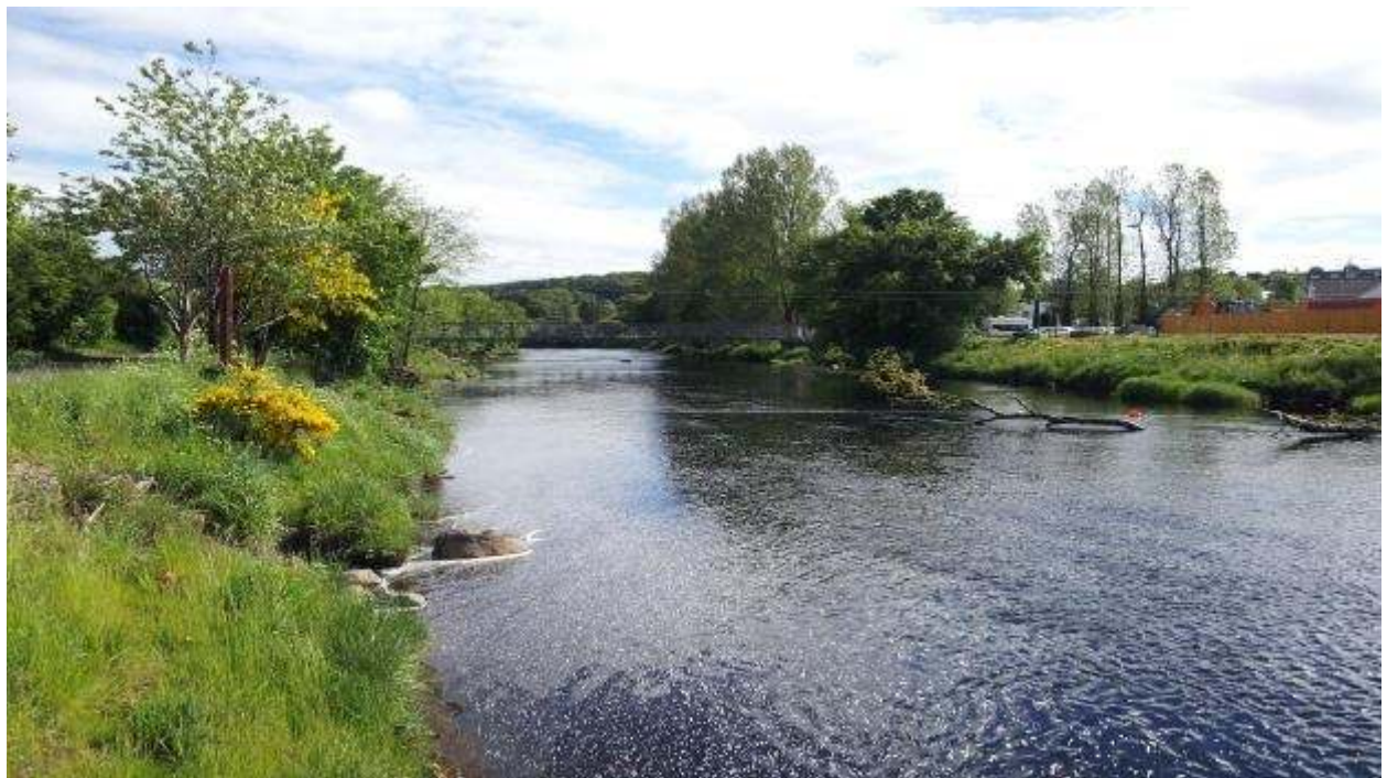
Photo – 13: River Cree – Upstream view of metal footbridge
