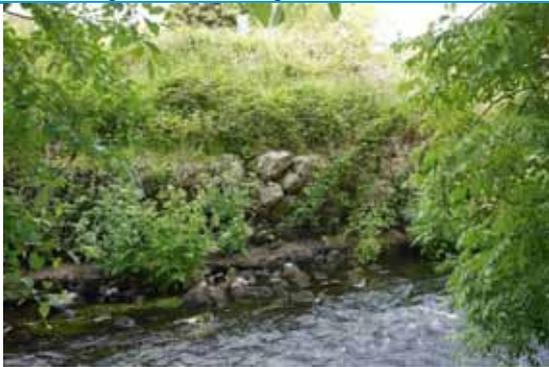
*Right bank rock armour and eroded concrete sill*
