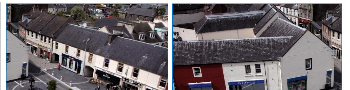
George Street and South Strand Street absence of chimneys in the roofscape around Castle Square
