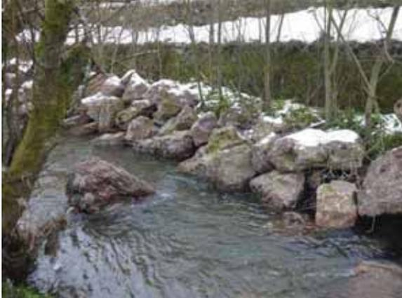
Photograph looking downstream showing dislodged boulder in channel bed
