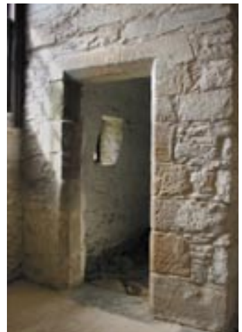
The entrance to the garderobe chamber. This was built during alterations to the hall in the mid seventeenth century.
