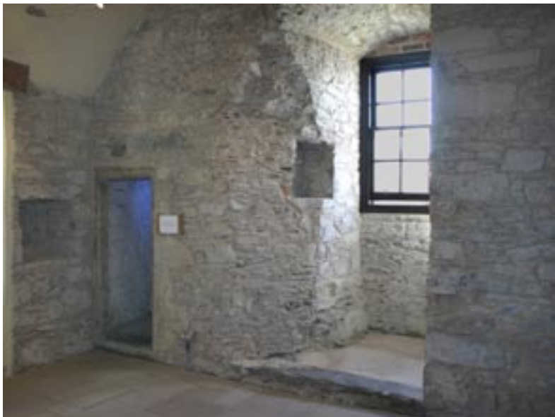
The west end of the hall. On the left is the entrance to the servants' staircase.
