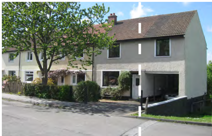
Above: This two storey extension to an end terraced house has been designed to continue the building and roof line of the existing terrace
