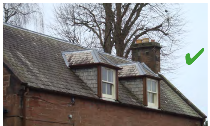
Below: Well designed dormer modestly scaled and within the roof plane
