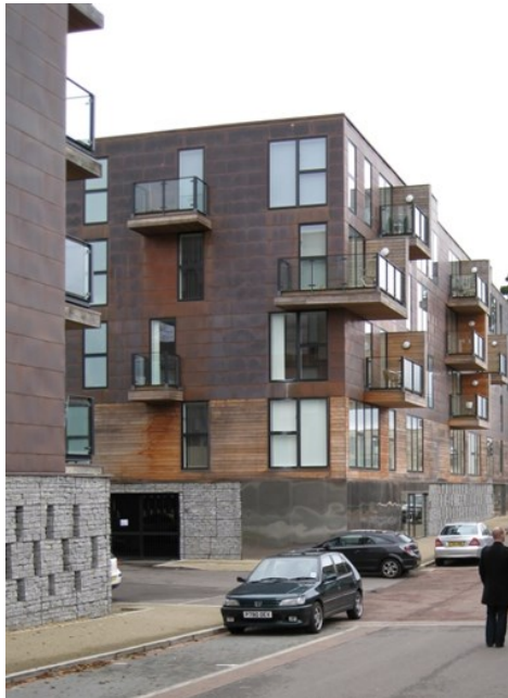
Above: an example of undercroft parking, Accordia, Cambridge
