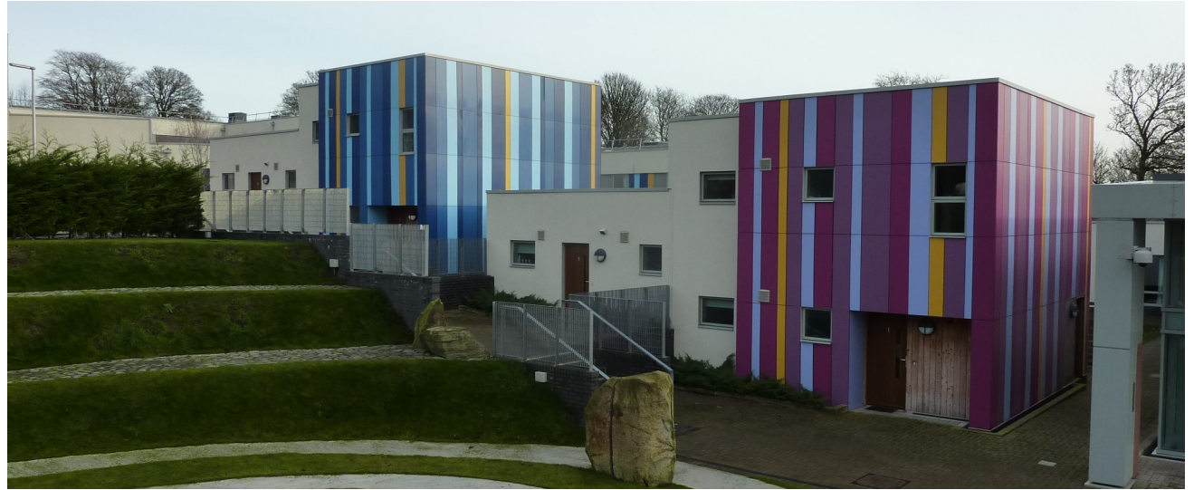
Above: Midpark Hospital, Dumfries which uses the sloping site to its advantage
