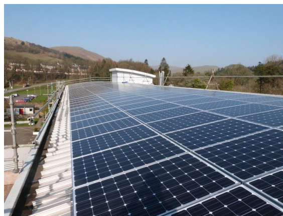
Above, solar panels at Langholm Academy
