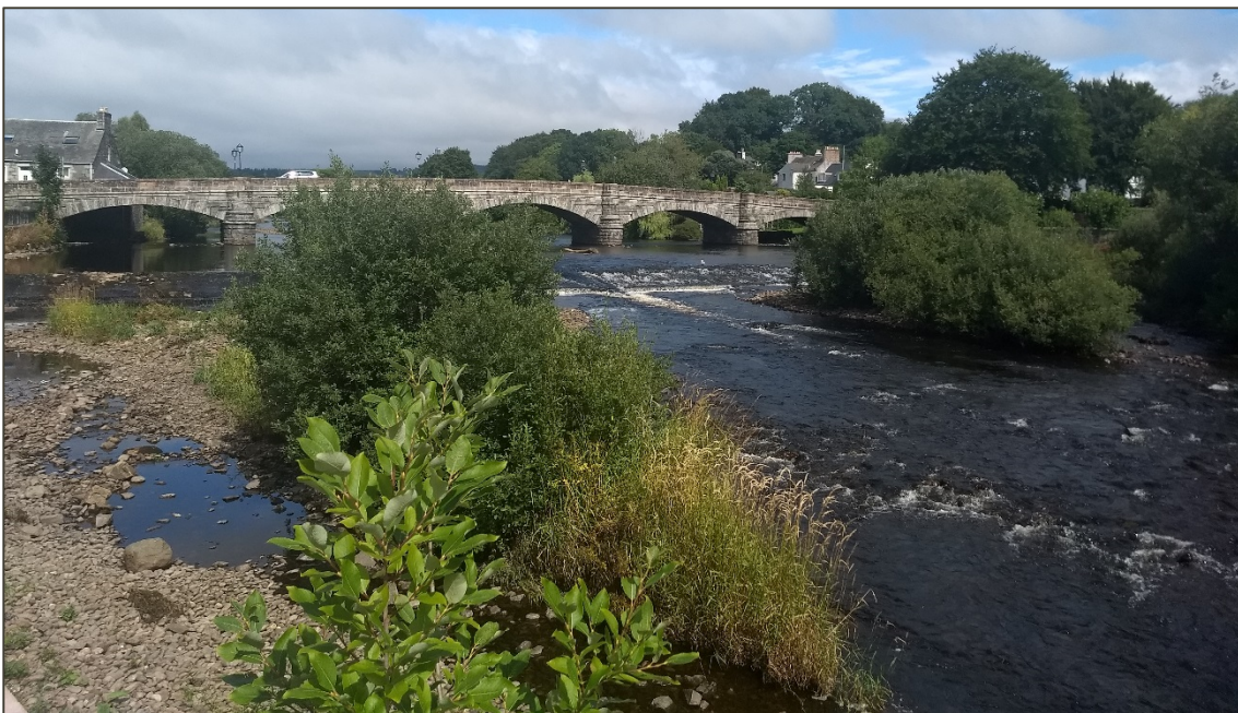
Figure 2. 7 Photo showing the weir on the River Cree downstream of the Cree Bridge. Deposition has occurred downstream of the weir.
