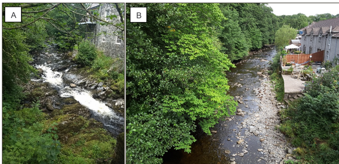
Figure 2. 9 Penkiln Burn (A) Bedrock exposed in channel at the Kirkland Farm footbridge. (B) Bank Reinforcement in gardens upstream of the Penkiln road bridge.
