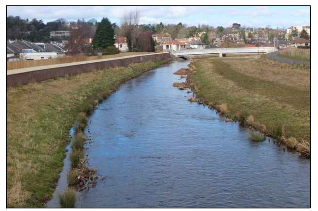
TYPICAL EXAMPLE OF BRICK FACED WALL (WATER OF LEITH, EDINBURGH)
