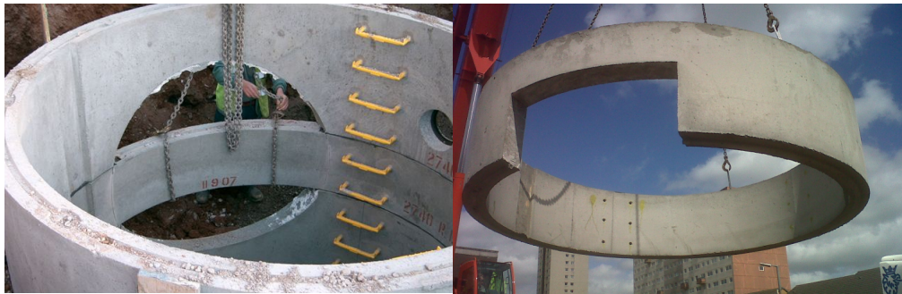
Figure 3.15 Typical large PC rings manhole (reference: http://www.cpm-group.com/products/drainage/sealed-manholes/ )
