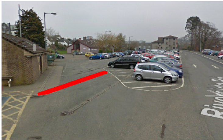
Figure 3.18 Photograph showing the location of the proposed Aco drain at the Area 16
