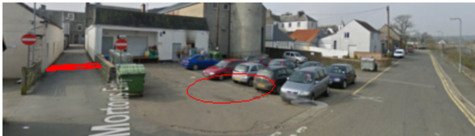
Figure 3.13 Photograph showing location of proposed drainage channel and the pumping station at Area 15
