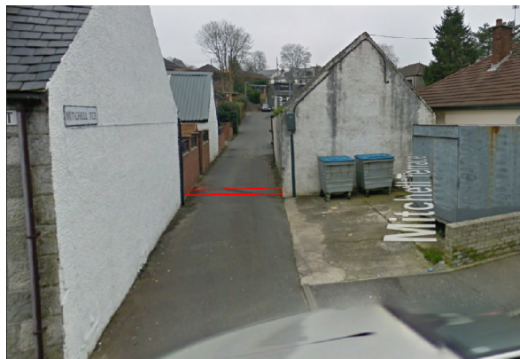
Figure 3.8 Photograph showing the location of the proposed heavy duty drain channel at Area 11
