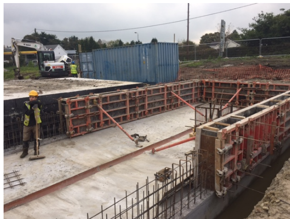
Figure 3.20 Typical in-situ reinforced attenuation tank (reference: http://trueformltd.co.uk/storm-water-attenuation-tanks/ )
