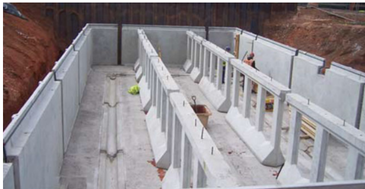
Figure 3.21 Typical precast concrete attenuation tank (reference: http://www.carlowprecast.co.uk/house-builder/stormcast-attenuation-system/ )
