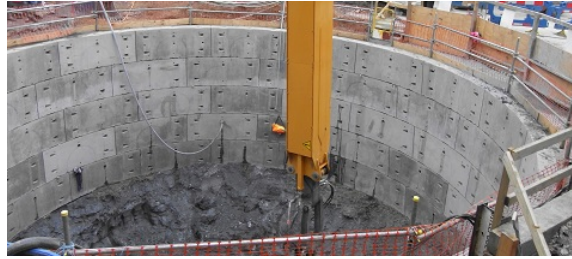
Figure 3.14 Typical Caisson manhole (reference: http://deltace.com/pages/caisson-shaft-construction.html )
