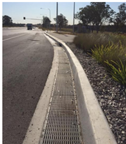
Figure 3.6 Typical drainage channel located at a kerblines of a road (reference: https://www.acodrain.com.au/news/drainage-products-camden-valley-way-upgrade.htm )
