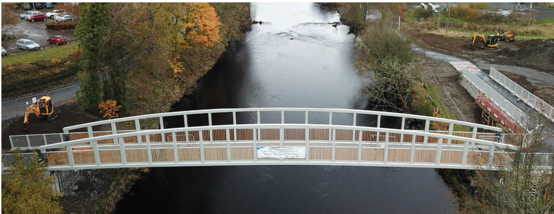
Figure 1-9 – New Sparling Bridge
