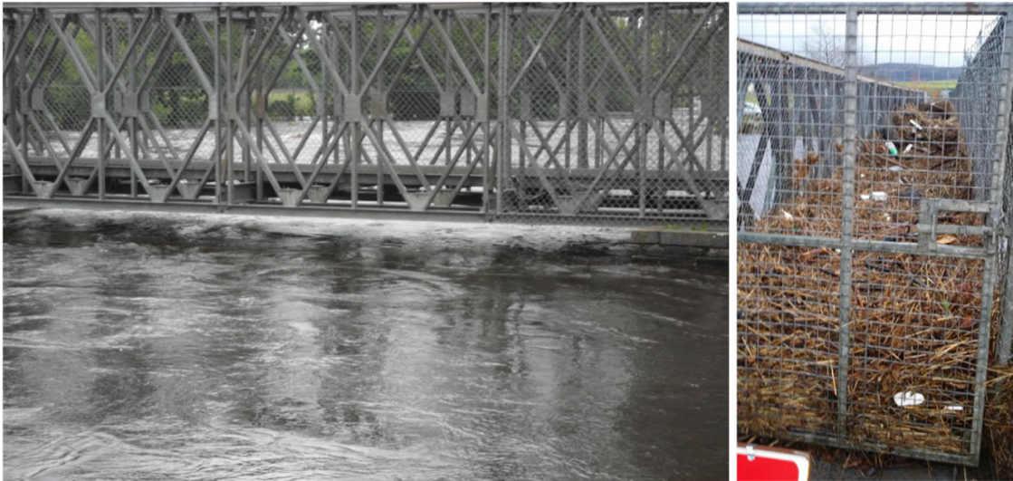
Figure 1-8 – Former Sparling Bridge design (left) and debris following flood event (right).
