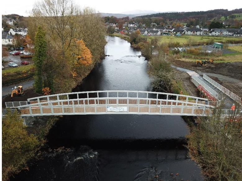
Bridge under construction
