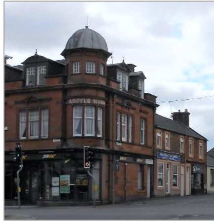
Argyle House 121 High Street
