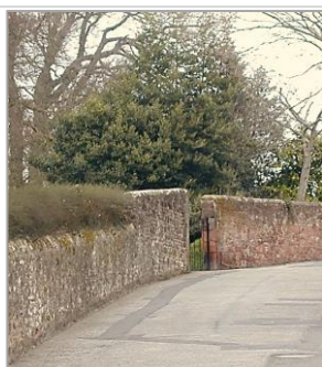
Walls on Bruce Street
