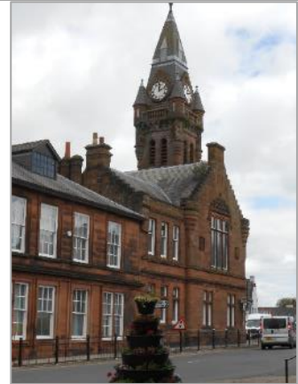
2,4 Battery Street & Town Hall
