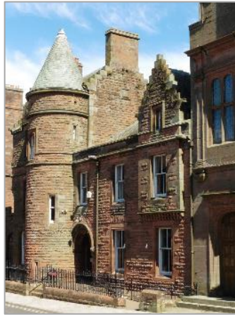
former Police Office
