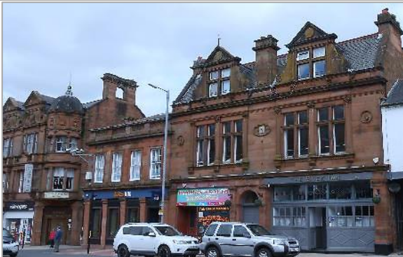
80 & 82 High Street and detail of 80 High Street
