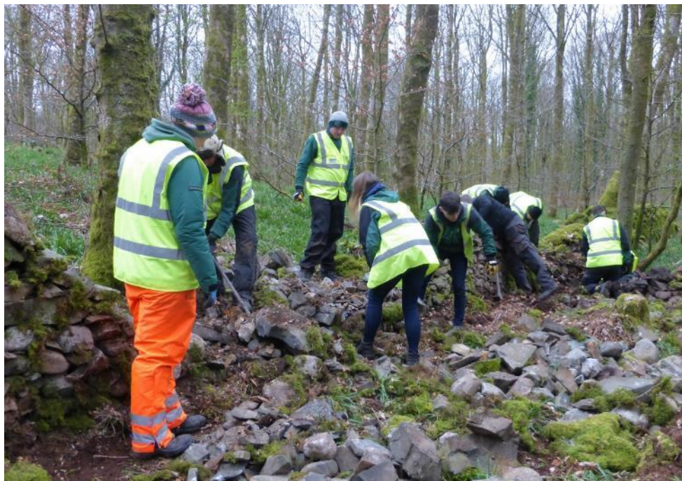
Apprentices clearing stone to re-build a wall
